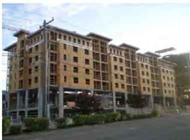
Figure 4 5-storey wood-frame apartment building on 2-storey concrete podium (2009), Seattle, Washington (courtesy: Sukh Johal c/o WoodWORKS/IBC)
