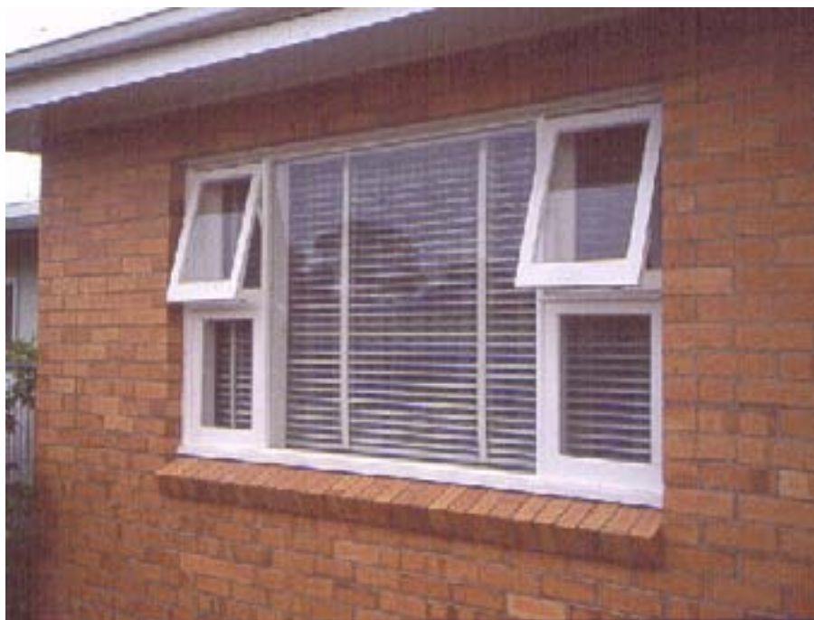
Figure 1.1: Eucalypt window 43 years old in Bairnsdale, with internal joints sealed prior to assembly, in excellent condition. For the purposes of the survey, this figure is considered to show one window.
