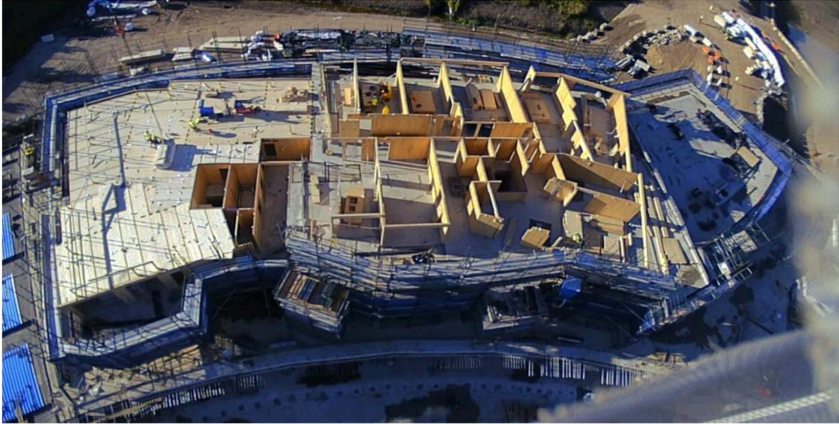
Figure 3: Overview of floor and wall installation on split Levels 4 and 5
