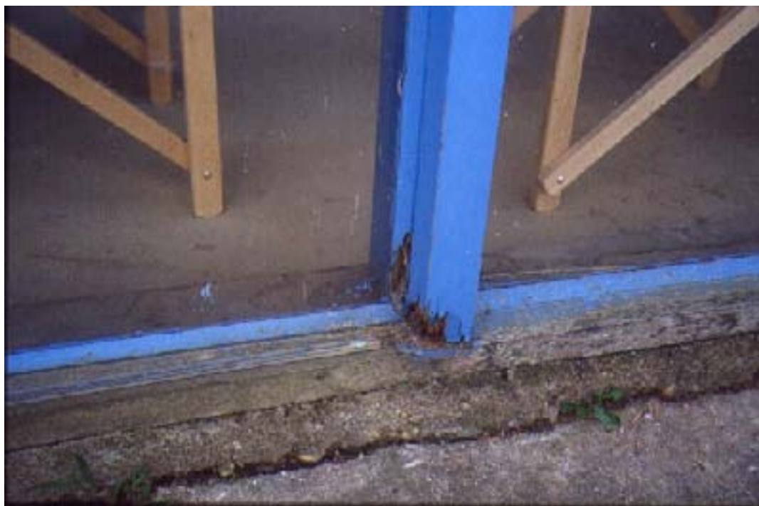
Figure 1.2: Brown rot in a 20 year old untreated western red cedar window.
